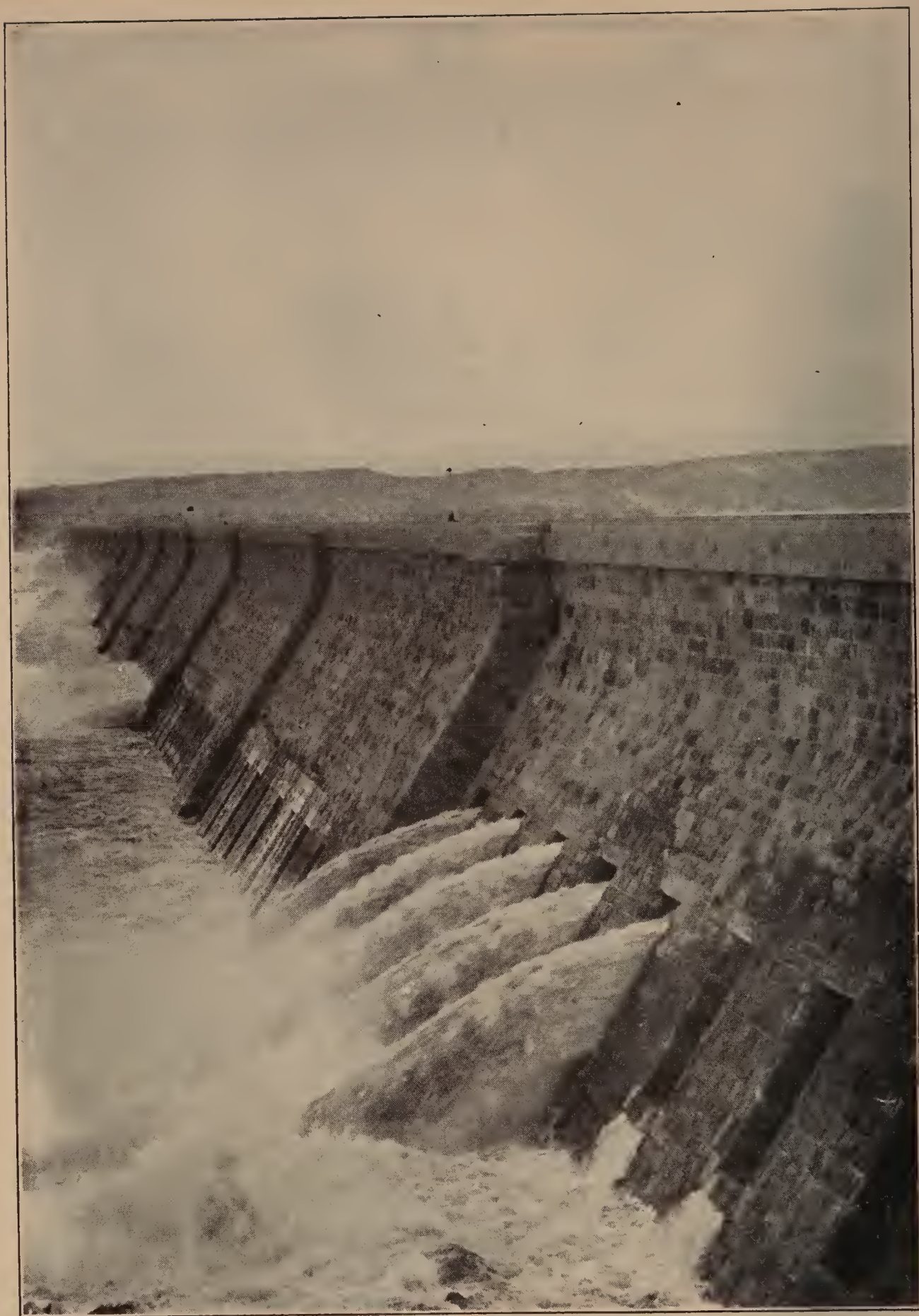
The Aswan Dam is a huge granite barrier a mile and a quarter long which now controls the waters of the Nile after centuries of alternate flood and drought, saves Egypt from famine, and adds millions of acres to her irrigable lands.
