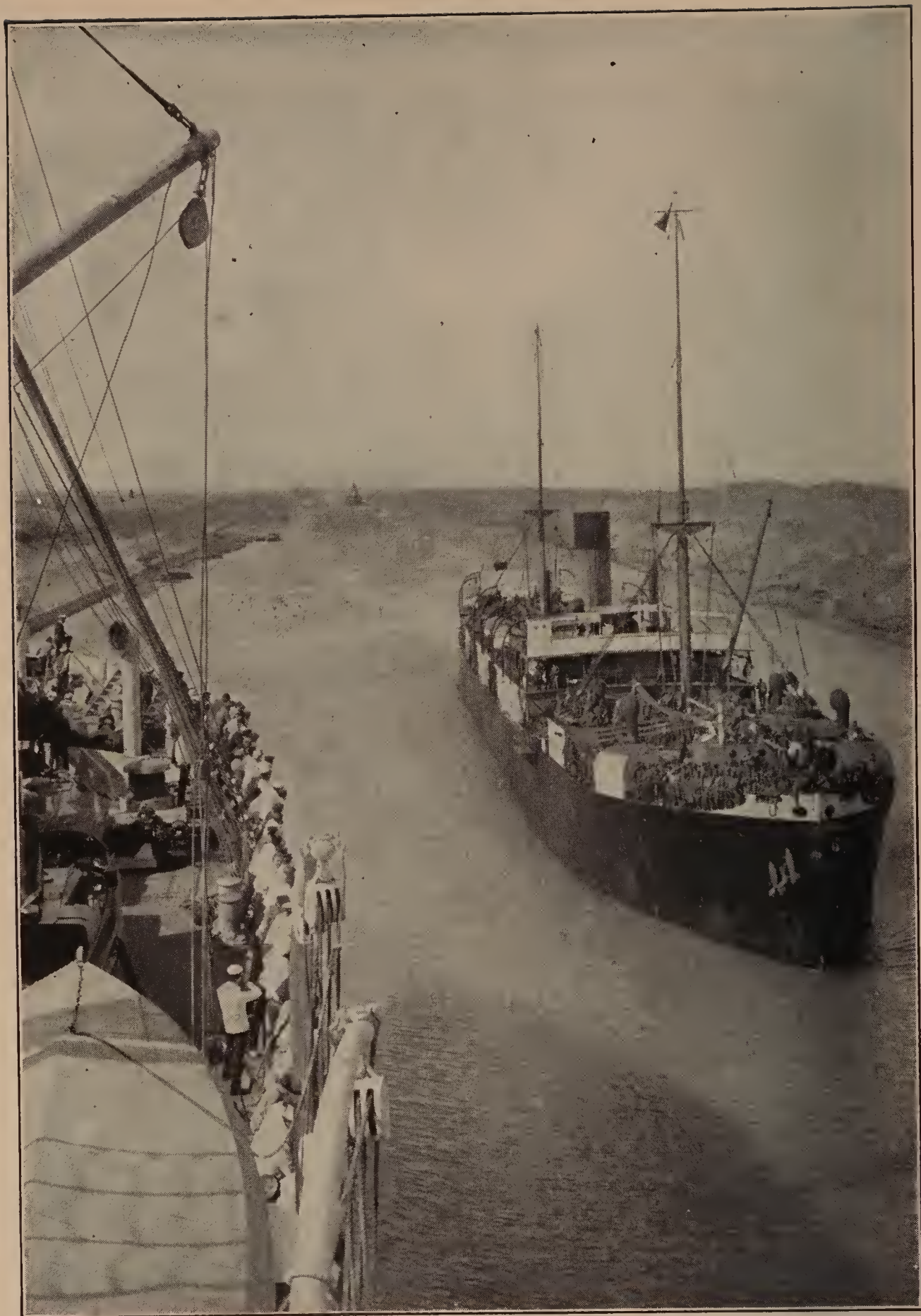
When two ships meet, one usually stops close to the bank and lets the other pass. In places the sides are lined with stones to prevent slides, and dredges are at work all the time keeping the channel clear.
