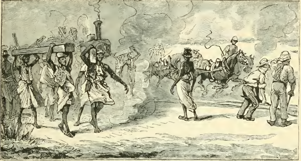
LAYING THE SUAKIM-BERBER RAILWAY.
