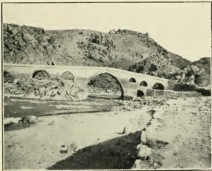
BRIDGE AT KEUPRI KEUI
