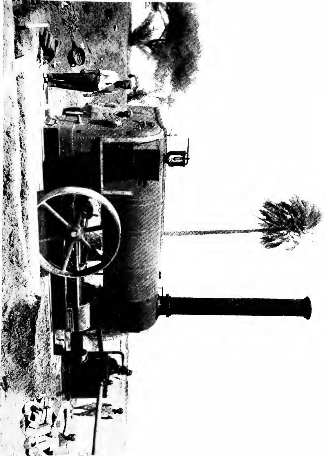
Under-type Pumping Engine at Turi Island—an Approved Pattern, adapted to Wood or Liquid Fuel.
