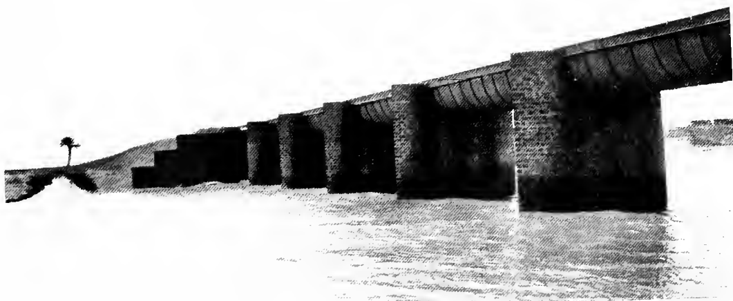
Trough Flume across Khor at Shambat.
