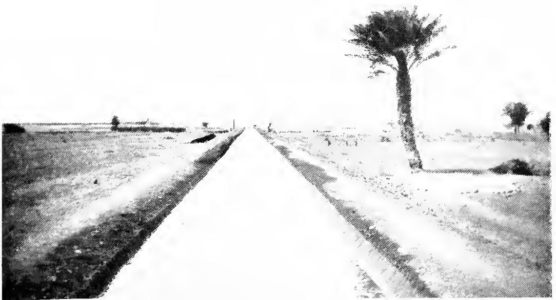
A Canal with Single Brick Lining after Three Years' Service, Shambat.
