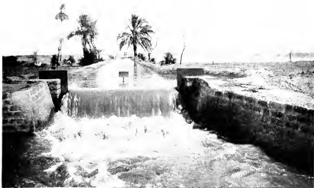
Measuring Weir at the Tuti Island Pumping Station
