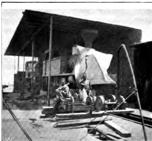
LOCOMOTIVE UNDER REPAIR, HALFA ARSENAL.
