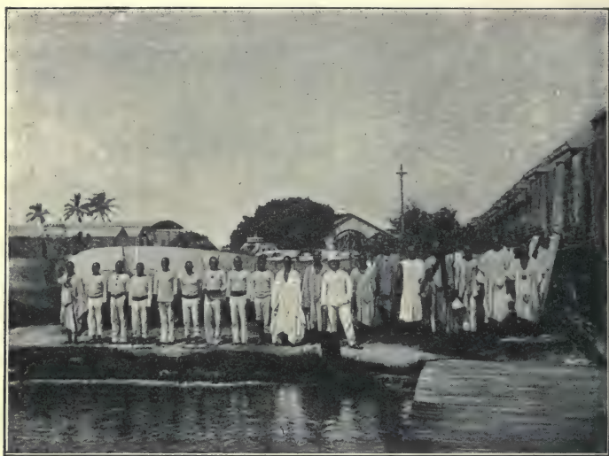
THE COOLIES ENGAGED AT ST. LOUIS.
