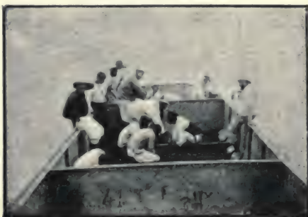
TIGHTENING THE BOLTS OF THE 'DAVOUST.'
