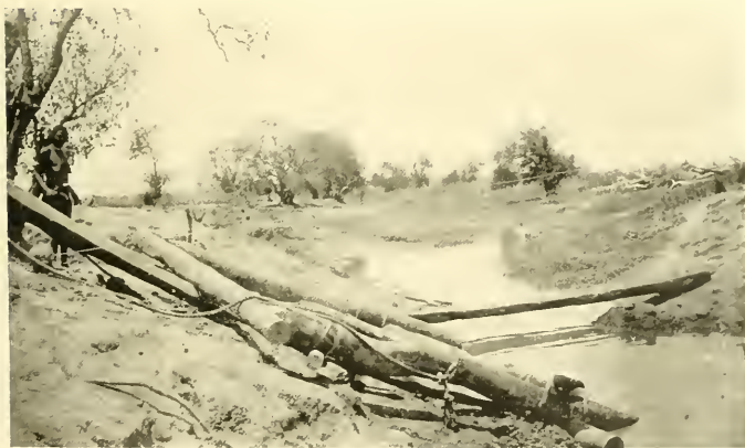
BRIDGE BUILDING. MAHOGANY BAULKS : TELEGRAPH WIRE : DOGS OF LOCAL IRON : AND SLIPS OF SPLIT PALM.
