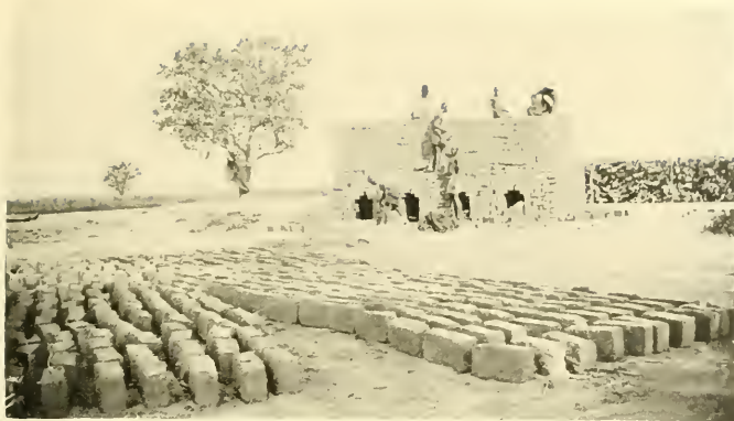
BRICK MAKING. THE FIRST KILN IN WAU
